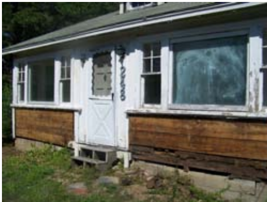
Michelle's home during renovations
